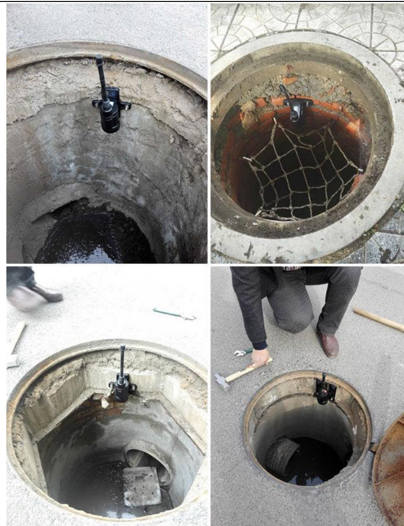
Manholes and WiiLSW sensors
