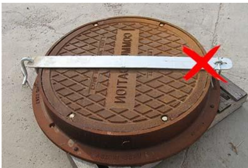
Manhole cover lock and protector.
