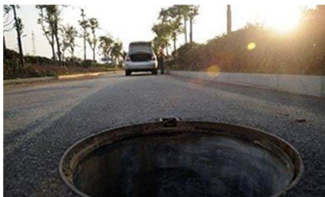
Manholes and manhole covers are everywhere.
